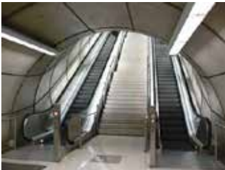
Picture 1.2.9.2. Example of escalators traveling in two opposite directions, a stop button attached to the stair in the center
