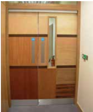
Picture 1.9.5.4. Example of the door which can be opened manually or pushed using the wheelchairs
