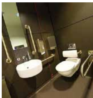
Picture 5.2.1.6. Sample of accessible unisex toilets with transfer on the right-hand side
