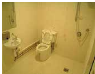
Picture 5.4.2.1. Sample of accessible shower with WC without grab rail and with external pipe.
