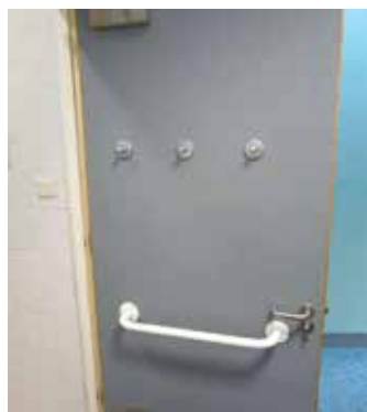
Picture 5.7.5.1. Sample of grab rails attached to the door
