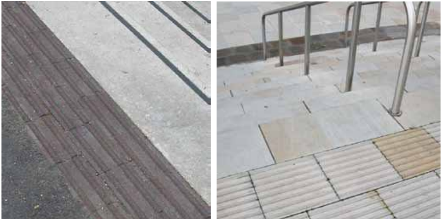
Picture 1.6.2.1. Example of signal surface at edge of stairs
