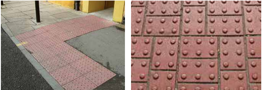
Picture 1.6.1.5. Example of red blister surfaces
