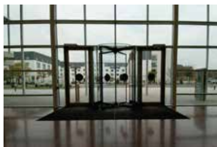
Picture 1.9.2.1. Example of two-wing automatic revolving doors
