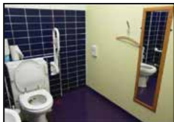
Picture 5.7.11.1. Sample of mirror attached to the wall in front of washbasin in toilet
