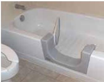
Picture 5.4.2. Sample of bathtub for persons with disabilities using wheelchairs
