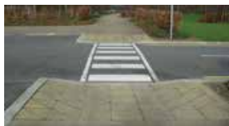
Picture 1.6.1.3. Example of brown surface at crossing points without traffic light
